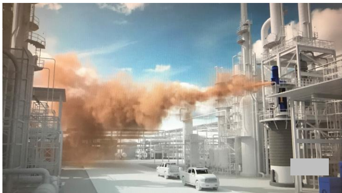
Figure 1: A computer-generated image depicting the horizontal release of ethylene vapour from EVAL Reactor 2's emergency pressure relief system
