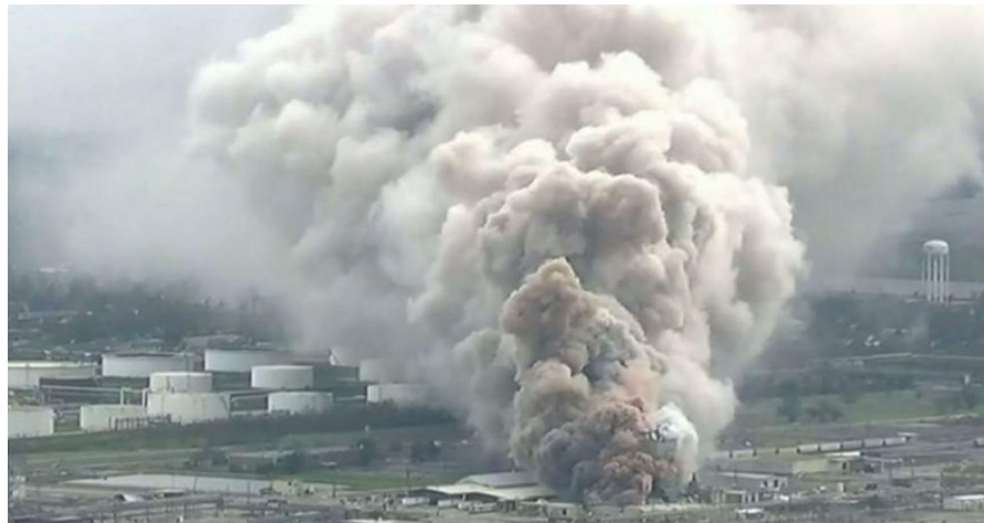
Figure 2: TCCA decomposition gases, including toxic chlorine, released from Bio-Lab Plant 4 after the building was severely damaged during Hurricane Laura and rainwater contacted the stored TCCA
