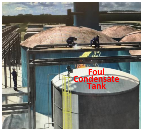
Figure 2: A computer-generated image depicting the hot work being performed on the pipework above the foul condensate tank
